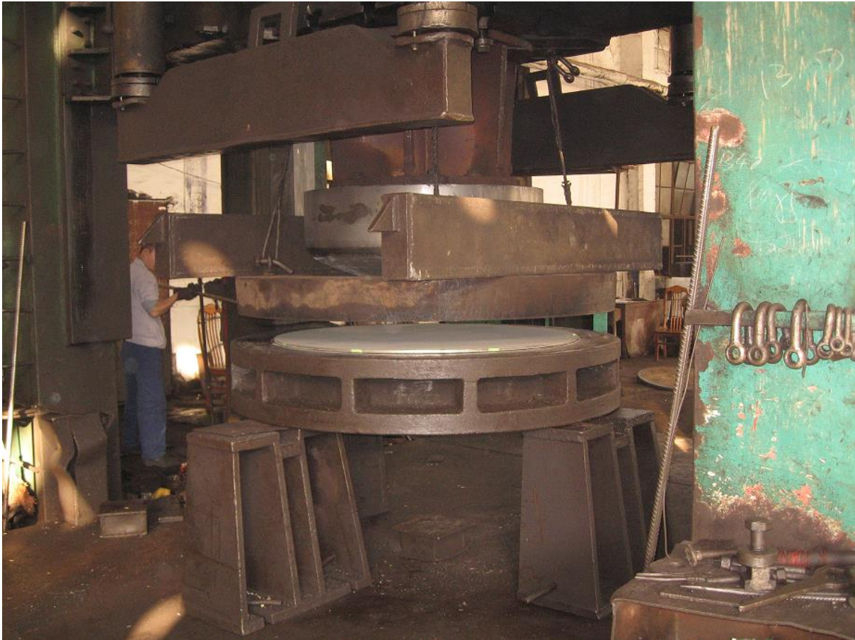
Procurement inspection – Check of the dish heads manufacturing conditions at Wuxi (China)
