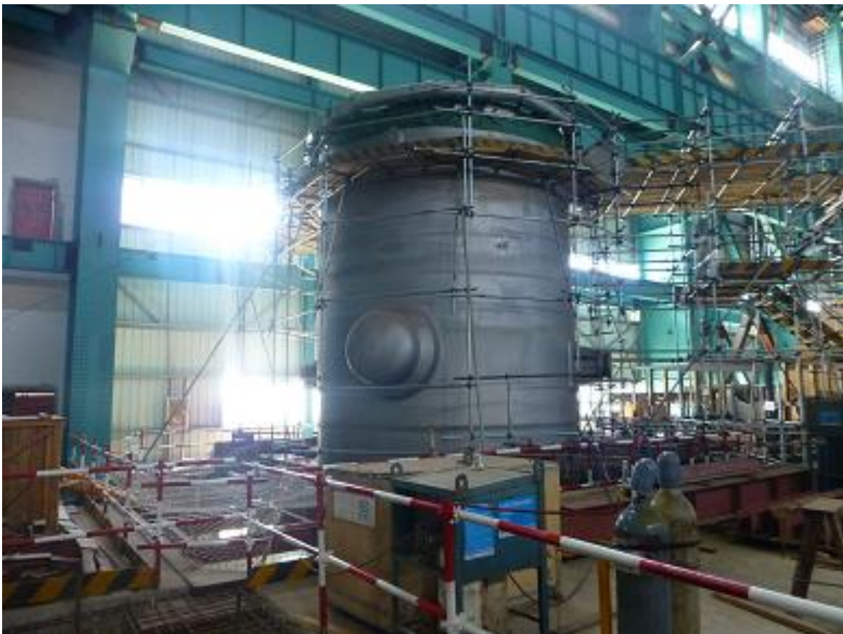
Site supervision – On site MSR installation supervision at Taishan (China)
